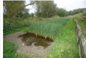
**Scope of Work:** ARM Ltd designed and built a 240m<sup>2</sup> horizontal flow reed bed treatment system to provide remedial treatment of groundwater by removing metals.
